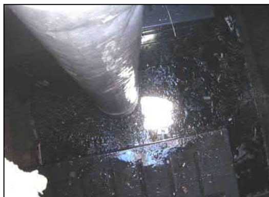
Removal of trash, sediment and debris.
