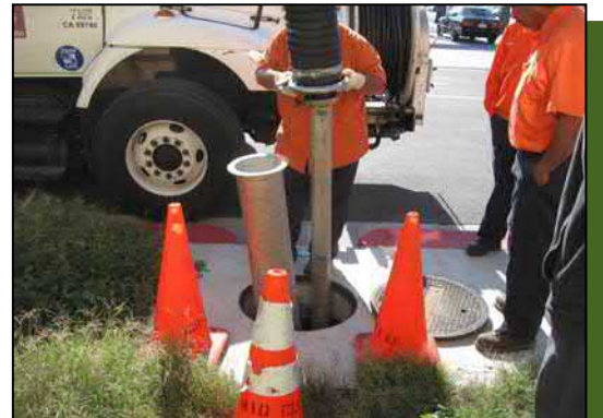
Insertion of vacuum hose into separation chamber.
