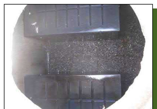
Fully cleaned separation chamber.
