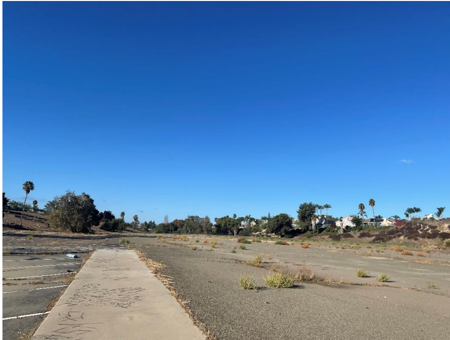
Figure 3. Parking lot, view facing west.
