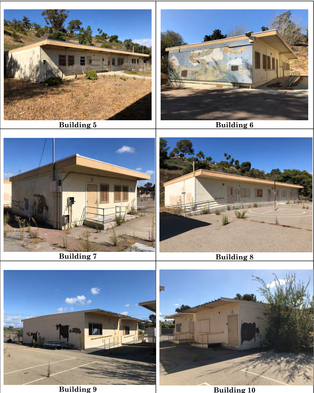
Figure 20. Current Views of Prefabricated Age Ineligible Buildings.
