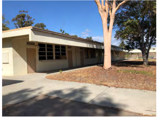
Unit B East Elevation
