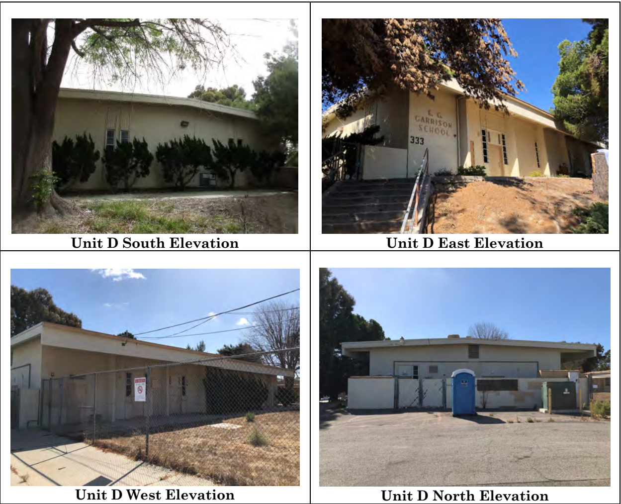
Figure 19. Current Views of Unit D.
