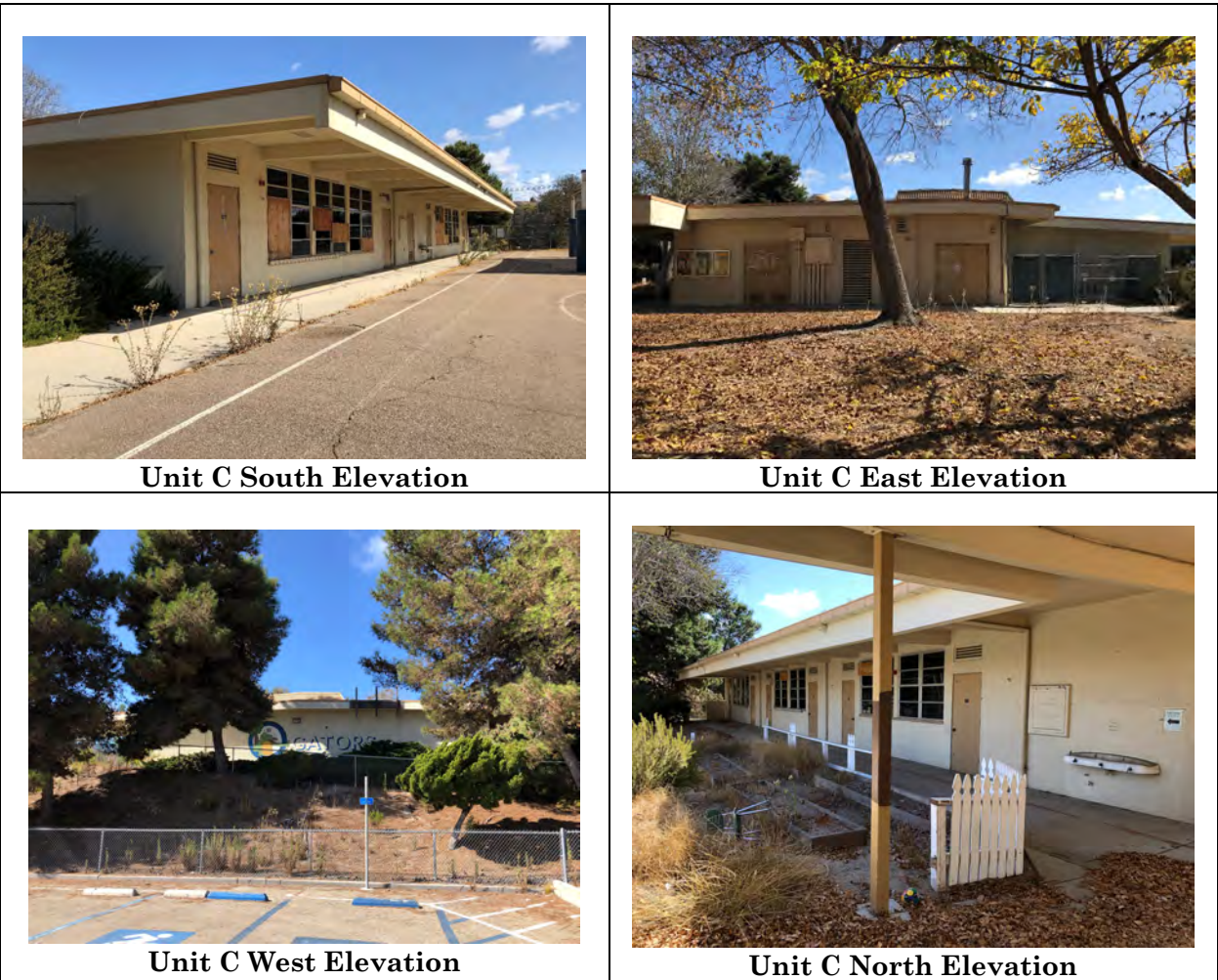
Figure 18. Current Views of Unit C.
