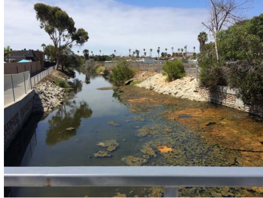
2 – Loma Alta Creek concrete-lined channel.
