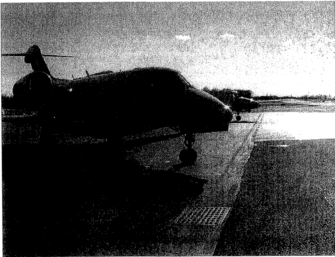
Flight line at Westchester County Airport – Ramp Storm Drain (Typical) AbTech UUF Catch Basin Insert Installed Under Grate
