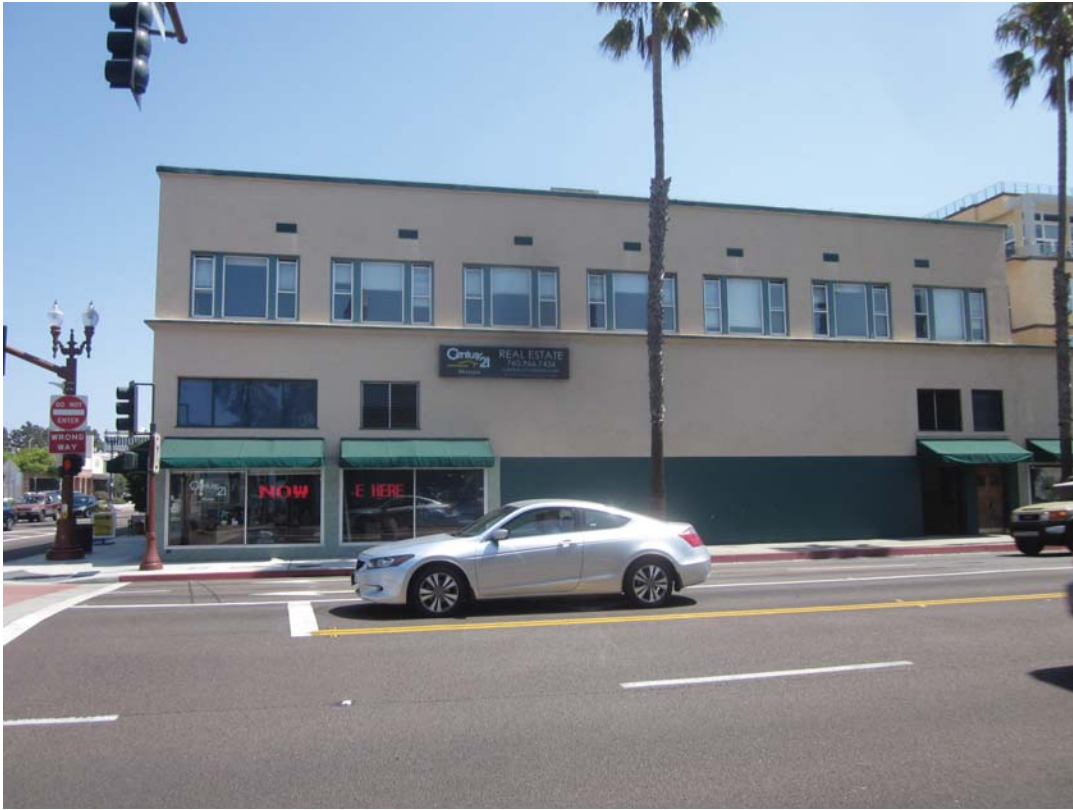
Overview of 501 Mission Avenue (view to east)
