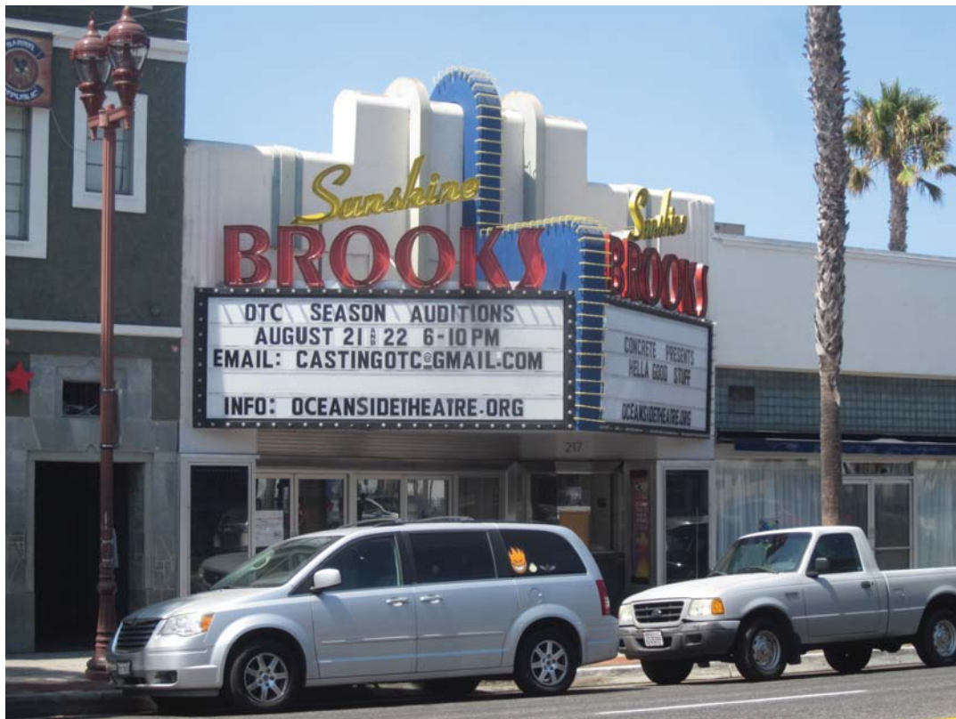
Overview of 217 Coast Highway (view to west)
