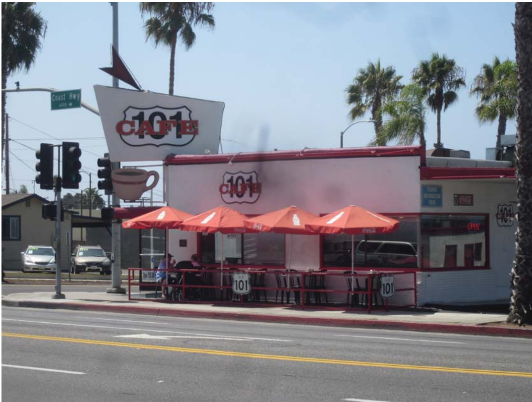
Overview of 631 Coast Highway (view to west)
