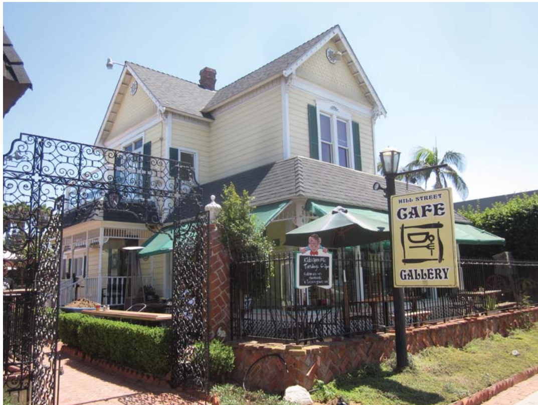
Overview of 524 Coast Highway (view to SE)
