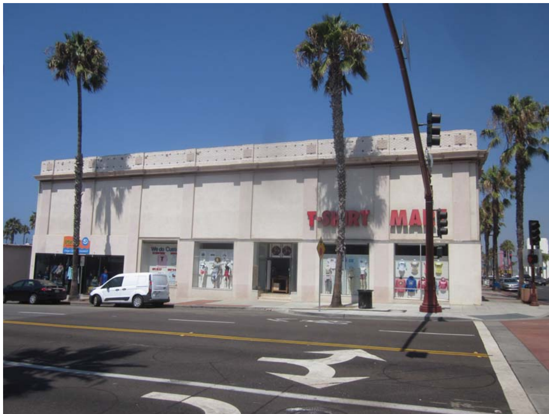
Overview of 201 Coast Highway (view to north)
