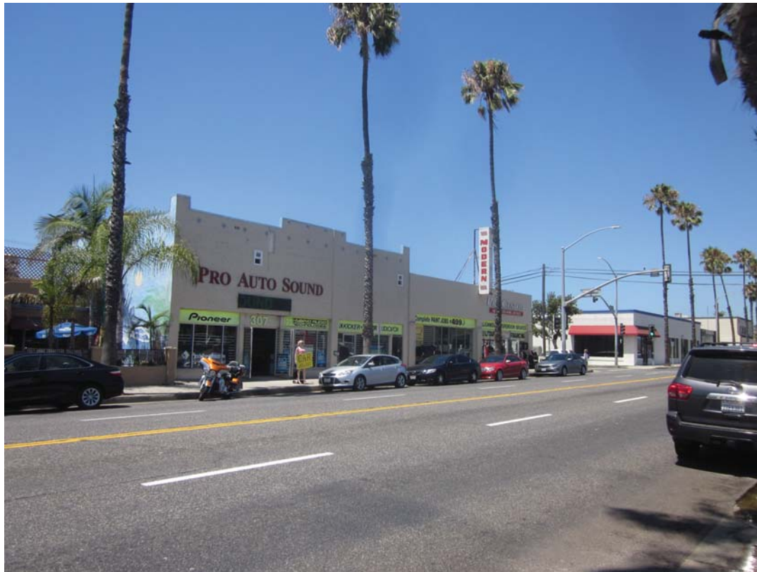
Overview of 301 Coast Highway (view to NW)
