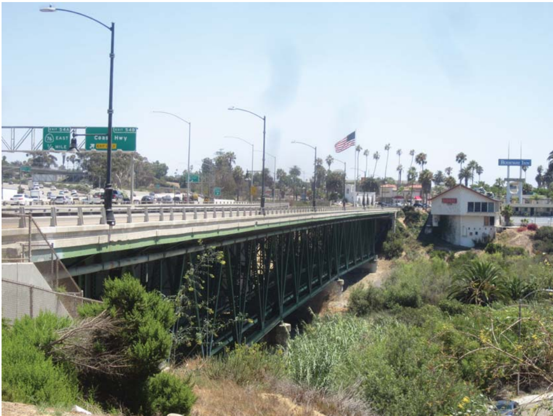
Overview of San Luis Rey River Bridge (view to south)
