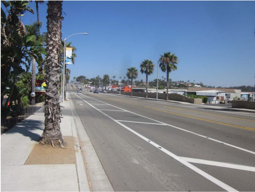
Survey conditions in central portion of complete street improvements (view to north)
