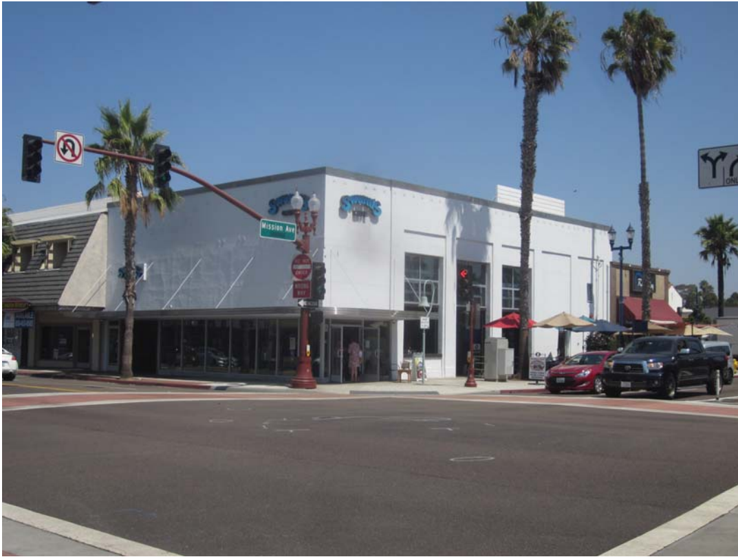
Overview of 202 Coast Highway (view to NE)
