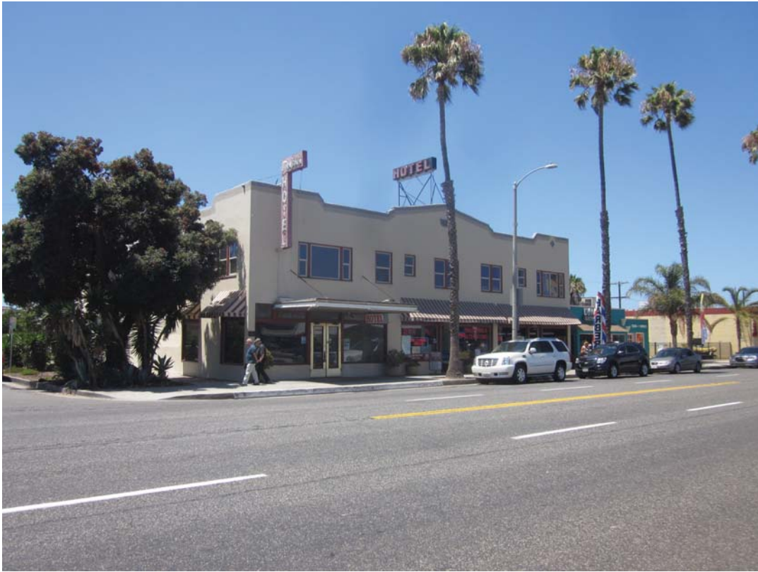
Overview of 133 Coast Highway (view to west)
