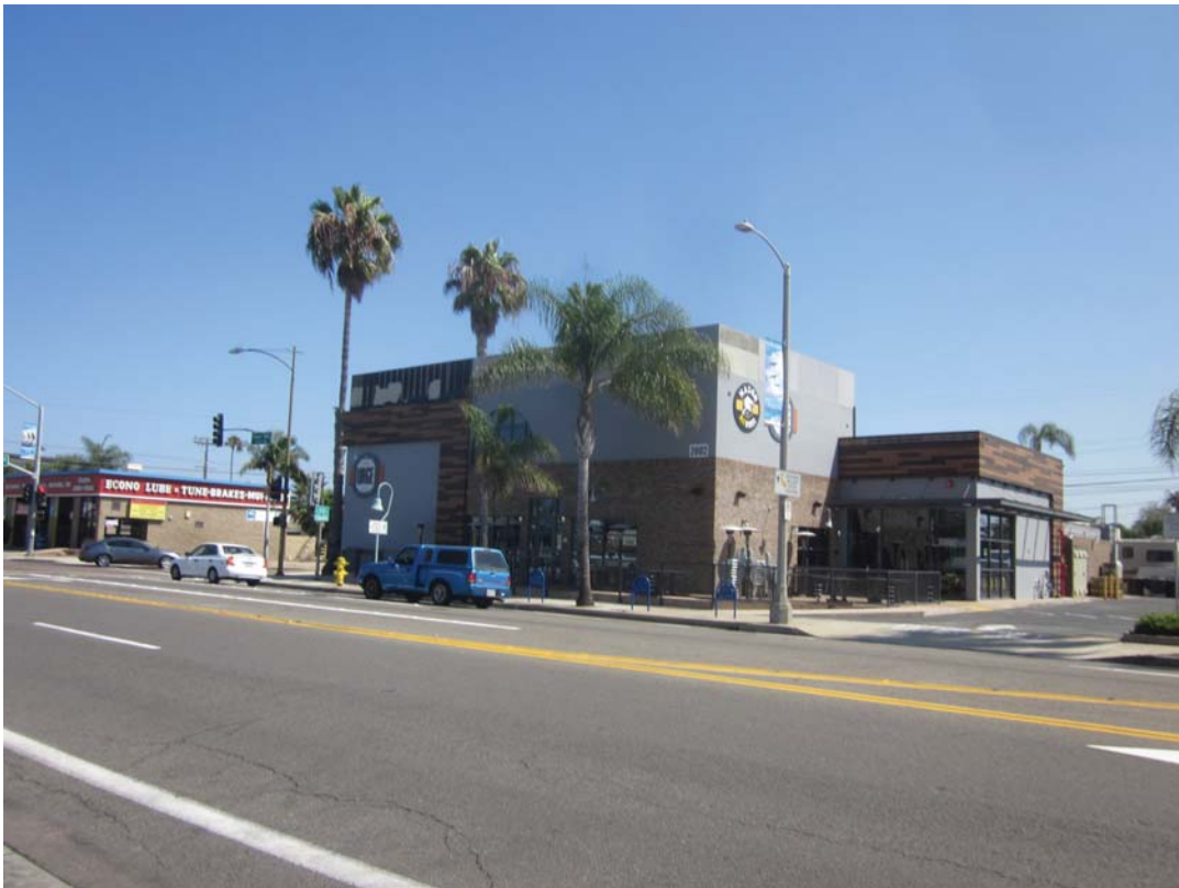
Overview of 2002 South Coast Highway (view to NE)
