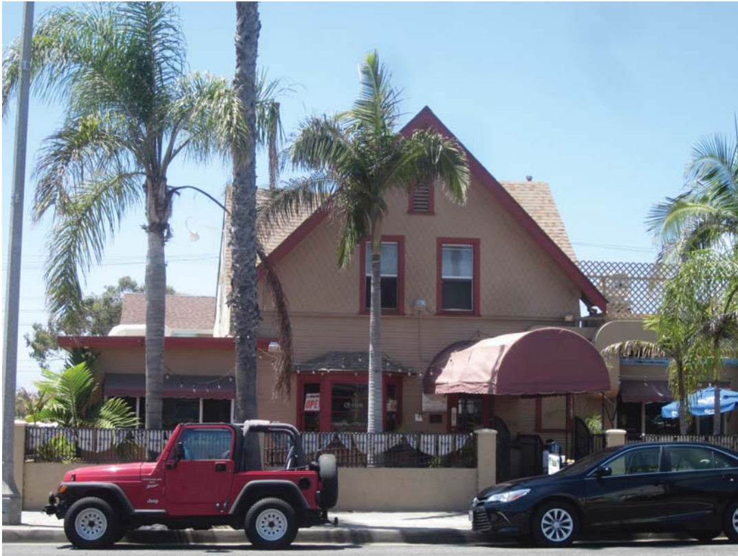
Overview of 309 Coast Highway (view to west)
